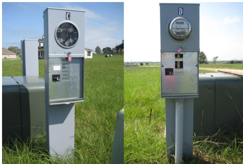
Left: Ready for hook-up
